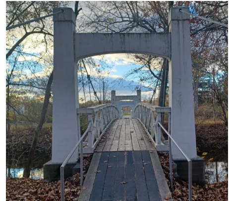
1937 Roebling Style Twin Foot Bridges - Lenape Park
