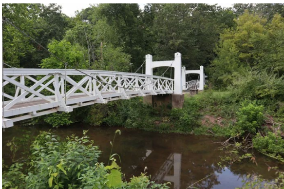
Pedestrian Foot bridge-Lenape Park
