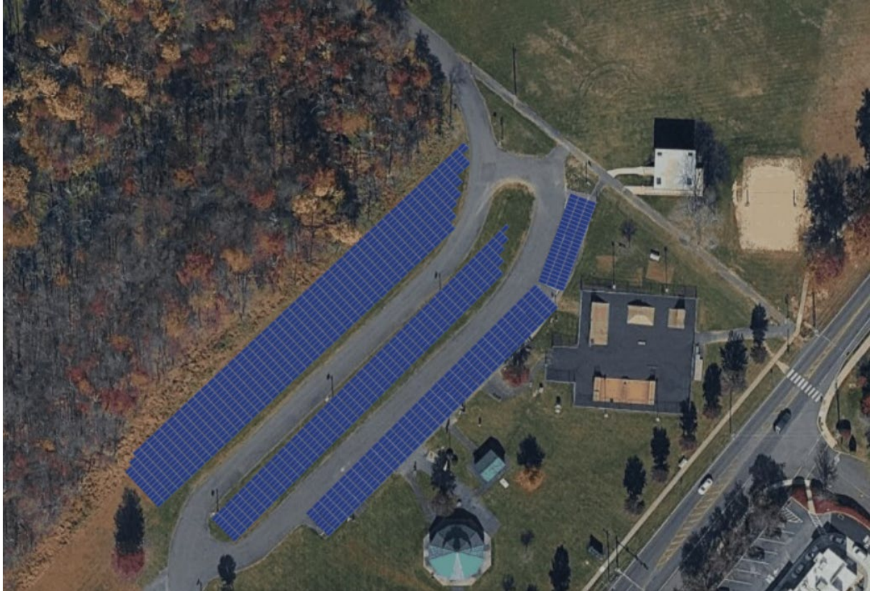
Lenape Park Parking Lot – 1106 Modules – 625W/module – 691.25kW DC – 500kW worth of inverters
