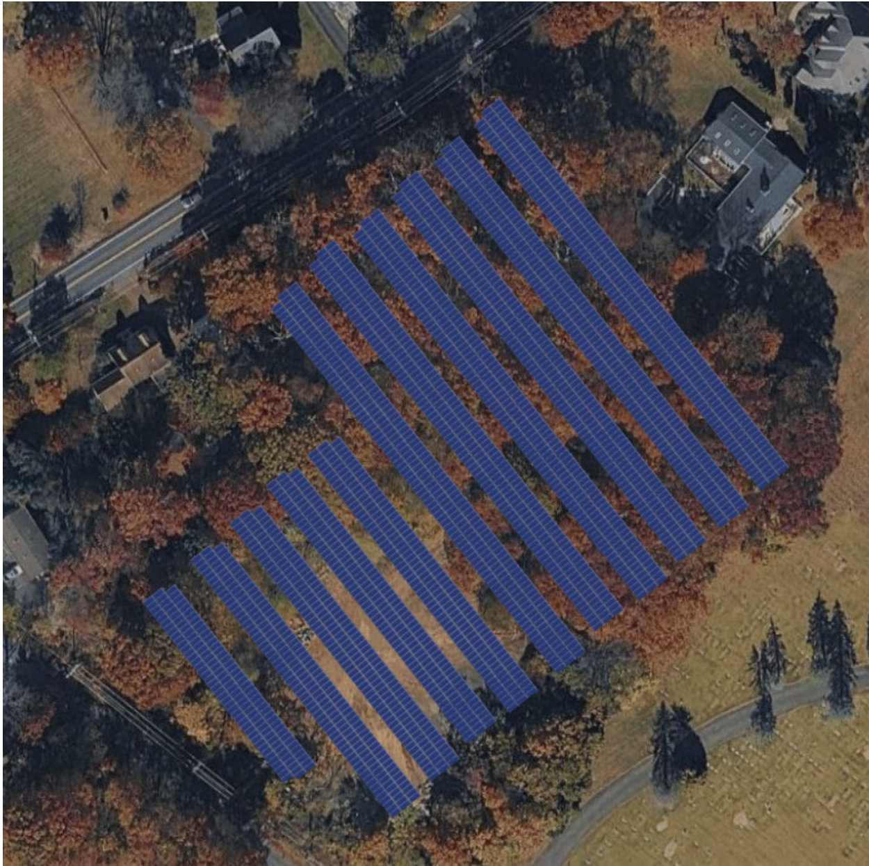
Landfill Site – 2385 Modules – 625W/module – 1490.63kW DC – 1100kW worth of inverters
