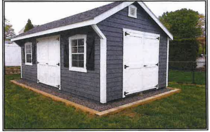
Crushed Stone pad with 1 Layer 6x6 perimeter
