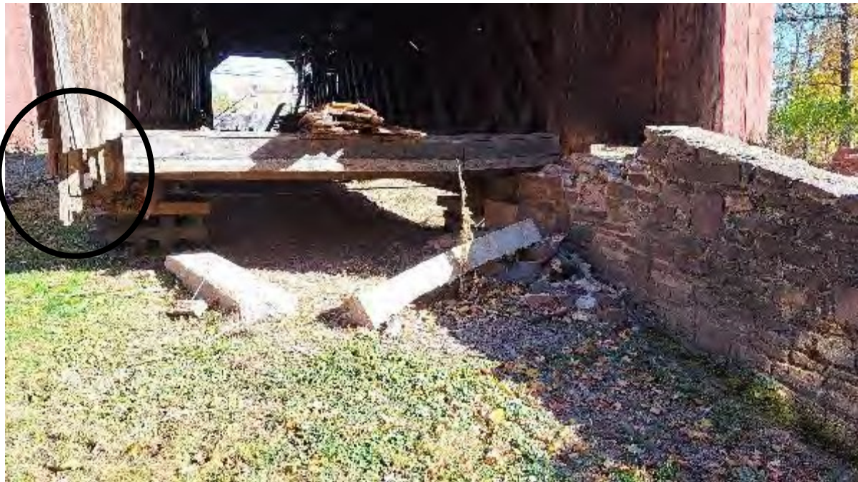
Image 4. Inspection report notes missing end beam and corner posts on the bridge’s North side (crushed post in circle)
