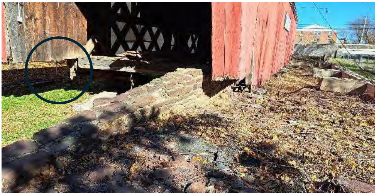
Image 3: Inspection Report Notes Missing Lower End Beam and Corner Posts on the bridge's North side (Crushed post in circle)
