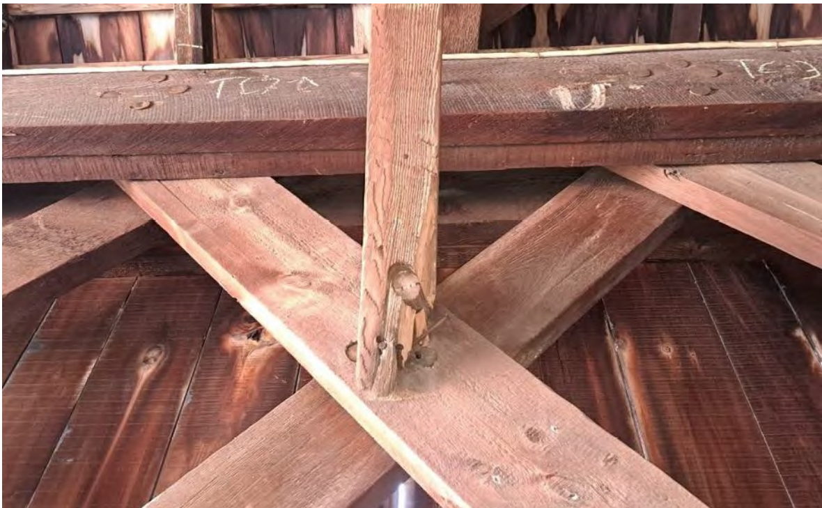
Image 5. Broken/cleaved dowel connection at knee brace KN2-S, WRD report
