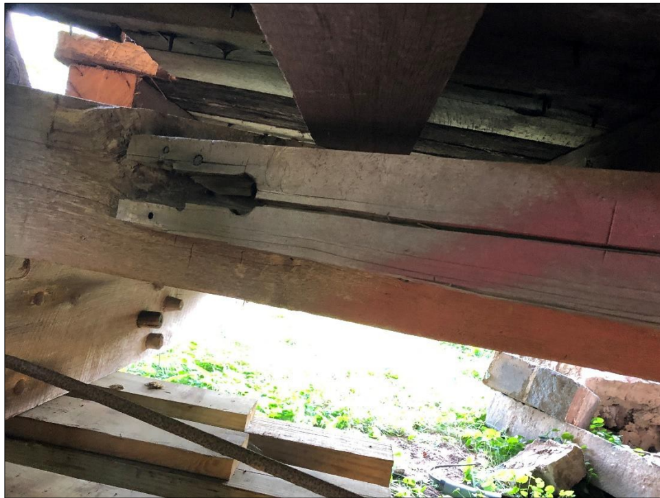
Photo 5 – View of the horizontal split at “X” bracing between FB1 and FB2. Note Missing Stringer S1.
