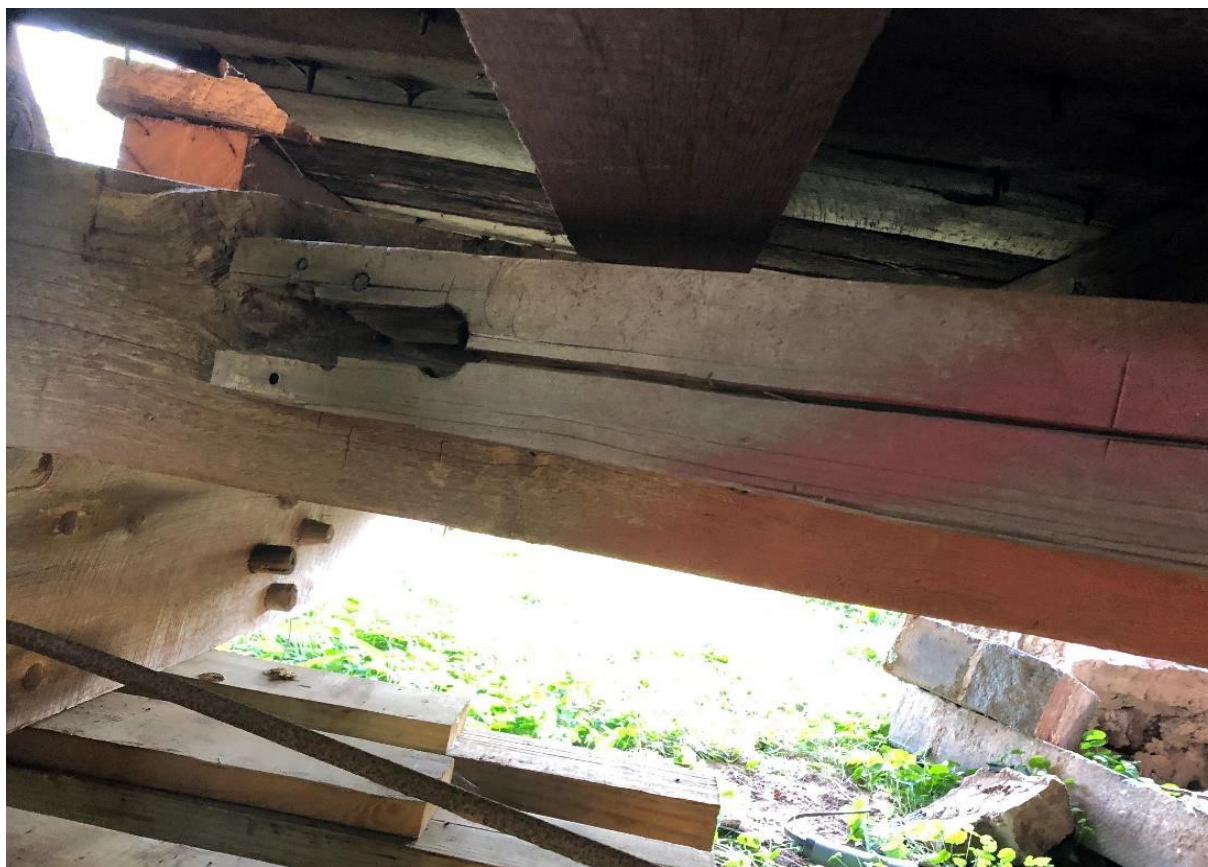
Image 1: Photo of a horizontal split at “X” bracing in Perkasio Borough engineer’s report
