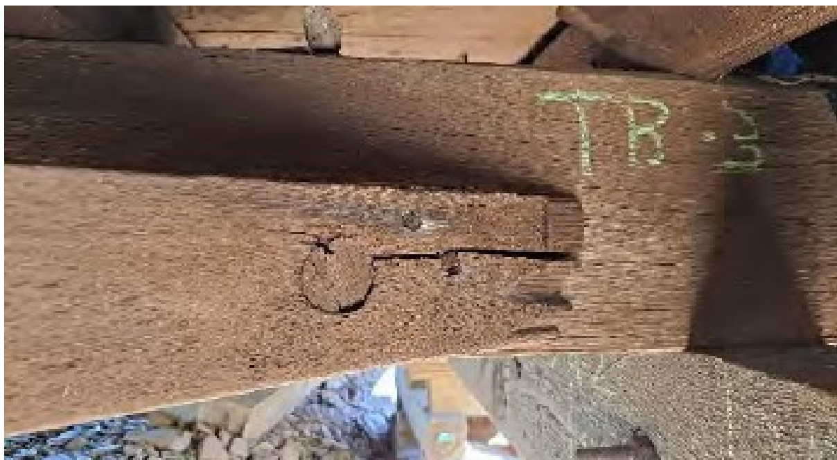
Image 2: Lower cross bracing dowel and spikes to transverse beam have cleaved, WRD report
