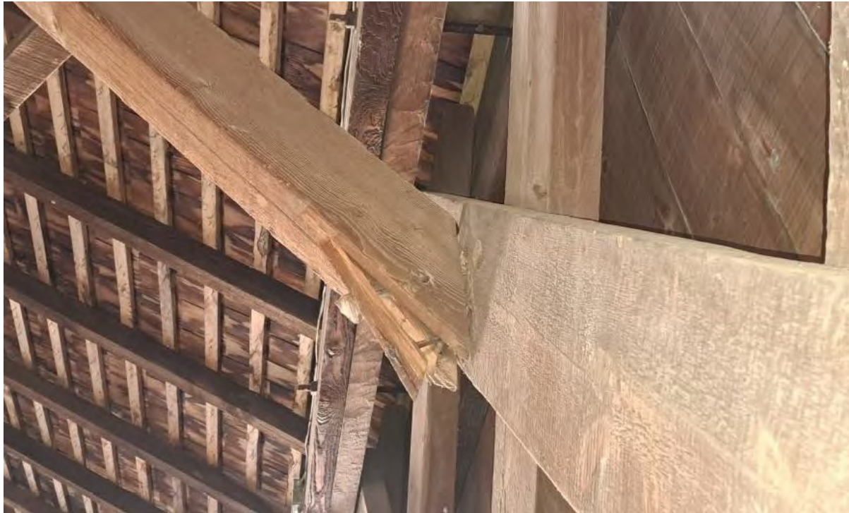
Image 6. Broken/cleaved dowel connection at knee brace, WRD report
