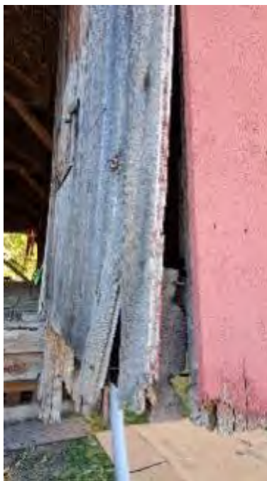
Figure 6-25: Abutment 1 North side wing wall with some section loss at the bottom.
