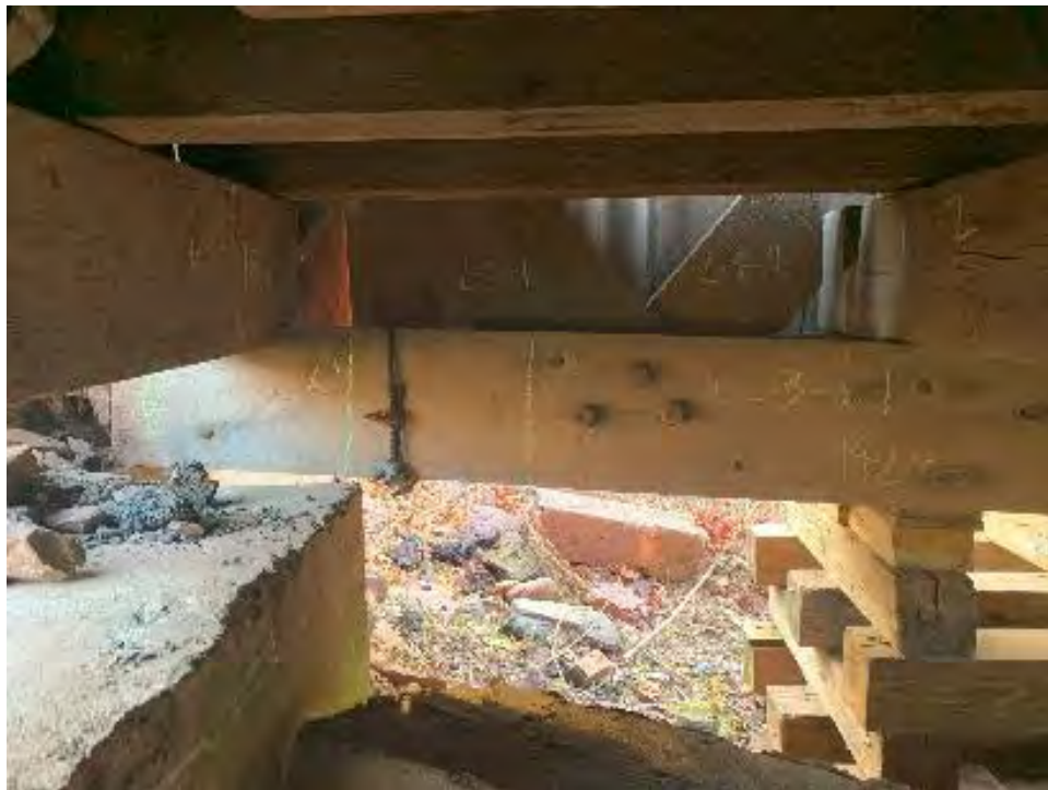
Figure 8-40: BC3A Abutment 1 end with temporary cribbing under bottom chords.
