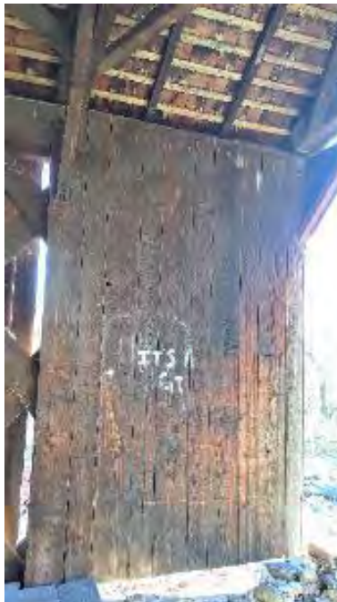
Figure 6-27: Abutment 2 South side wing wall internal view of siding.
