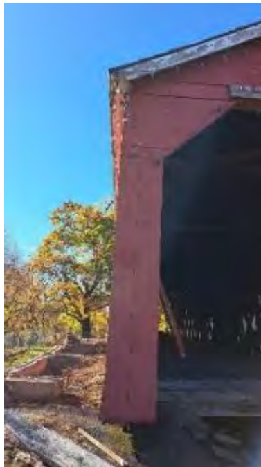
Figure 6-19: Abutment 1 South side front view of siding in fair condition.
