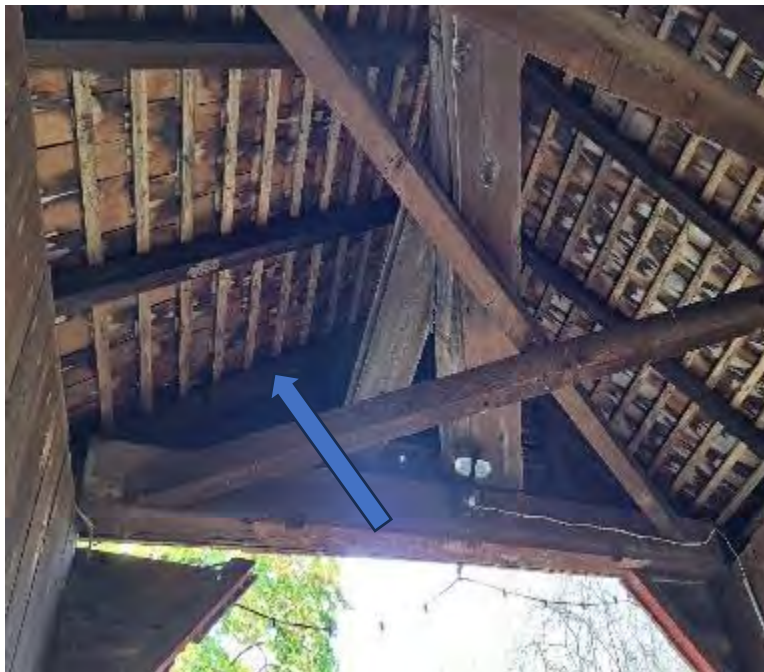
Figure 1-5: Abutment 2 Truss rafters, could not access the end near wing walls.
