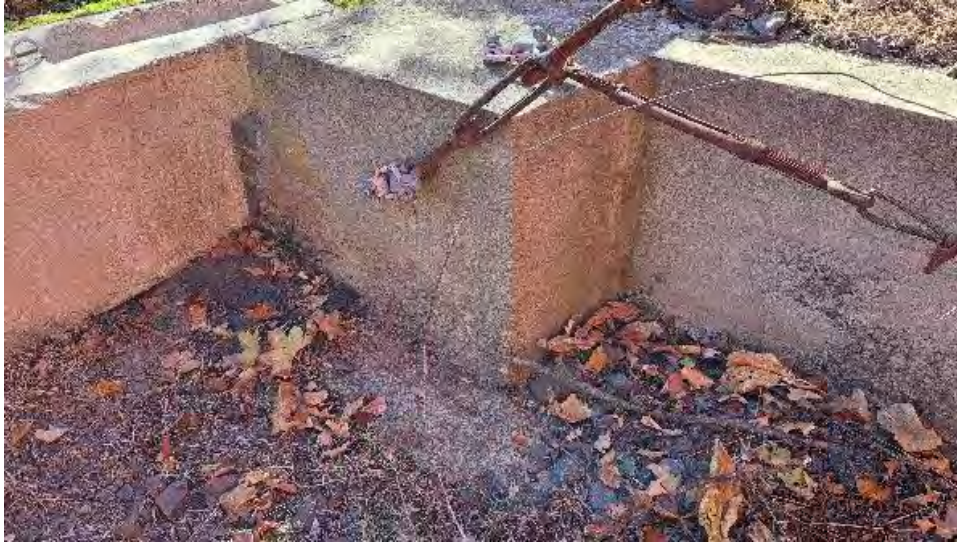
Figure 10-17: The mass concrete foundation at AB2 appears to be undamaged.
