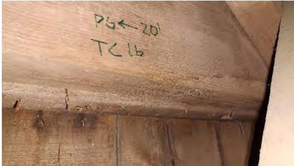
Figure 8-8: TC1B splice located 20-feet from post P6.
