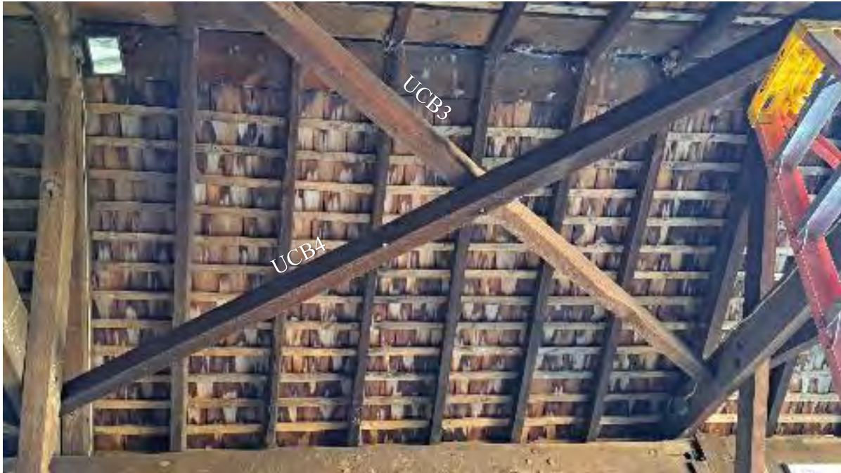
Figure 7-9: UCB3 / UCB4 in fair condition.
