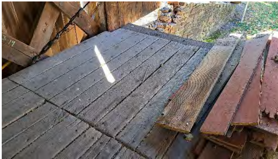
Figure 9-20: Floor decking Span 9, South side.
