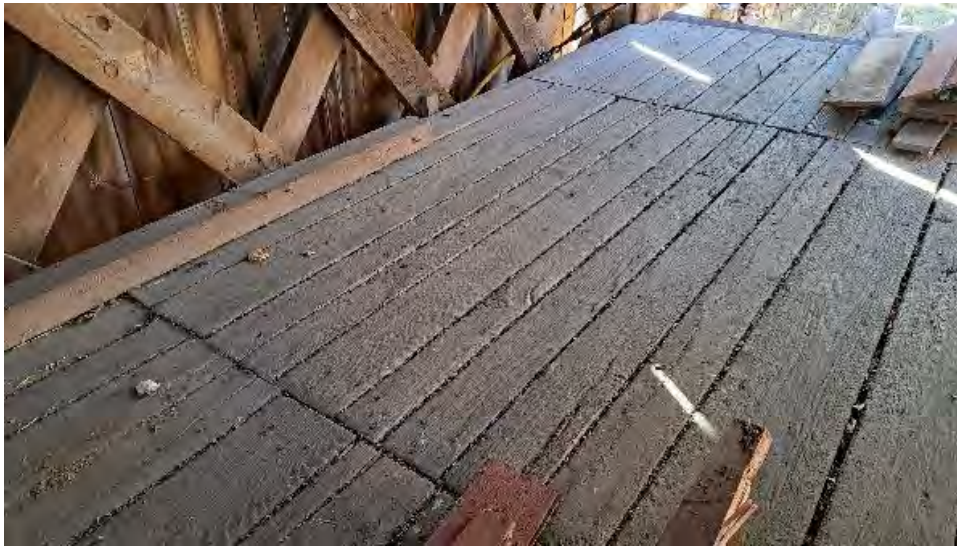
Figure 9-18: Floor decking Span 8, South side.
