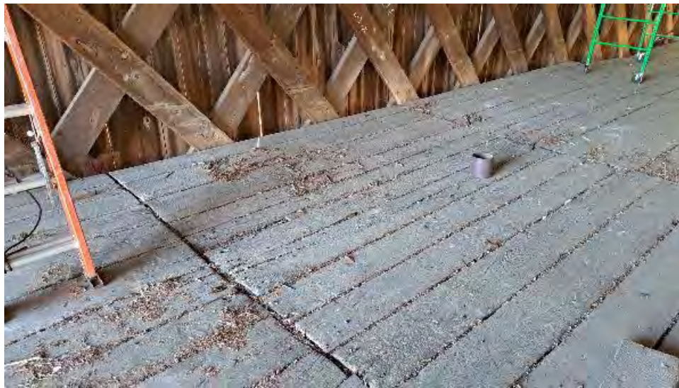
Figure 9-6: Floor decking Span 3, South side.
