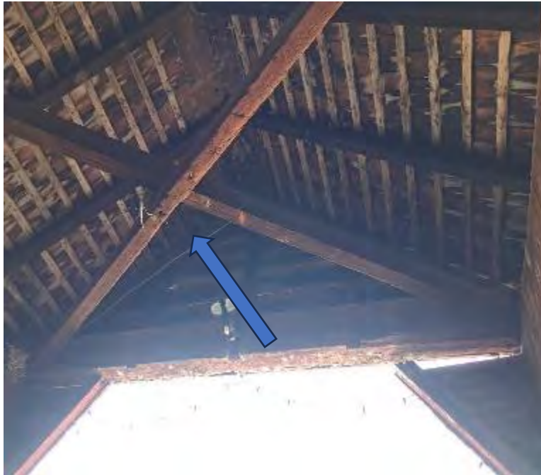
Figure 1-4: Abutment 1 Truss rafters, could not access the end near wing walls.
