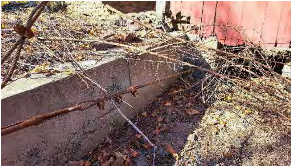
Figure 10-18: The mass concrete foundation at AB2 appears to be undamaged.
