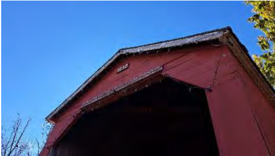
Figure 6-18: Abutment 1 front view of siding in fair condition.
