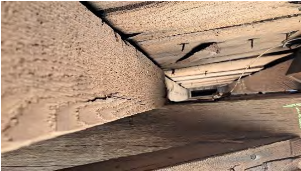
Figure 9-127: Joist J3-7 is continuous with J4-7.
