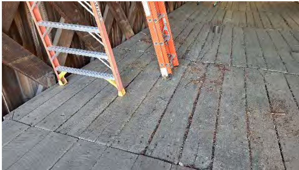
Figure 9-4: Floor decking Span 2, South side.
