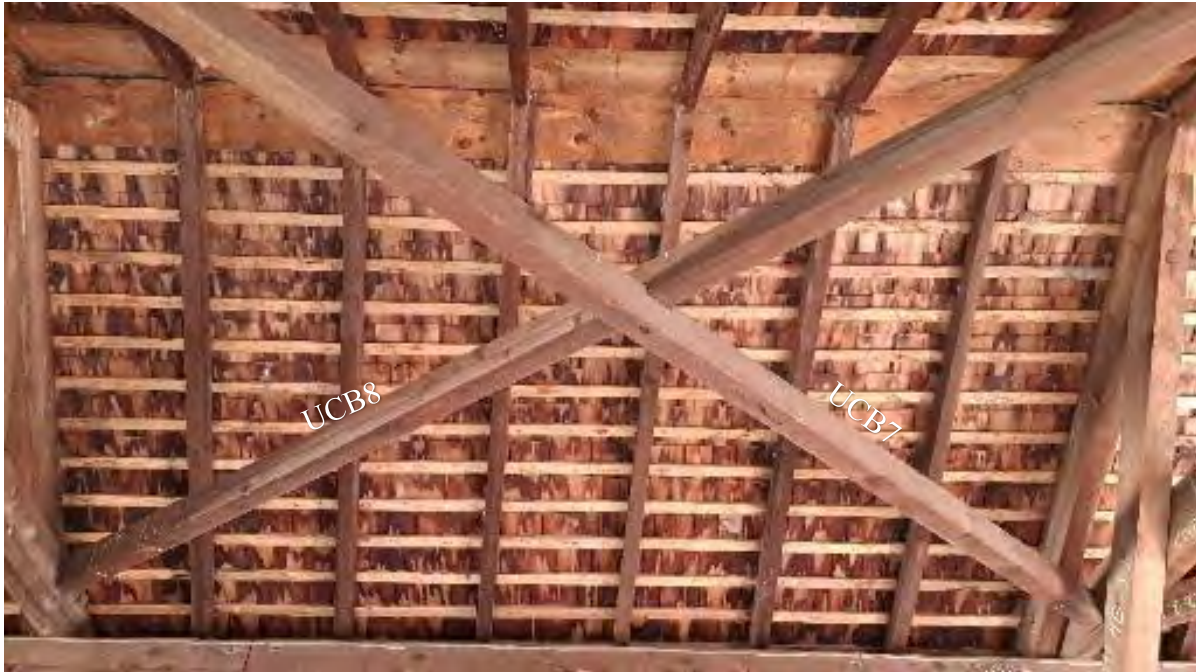
Figure 7-11: Upper cross braces UCB7 and UCB8 are in fair condition.
