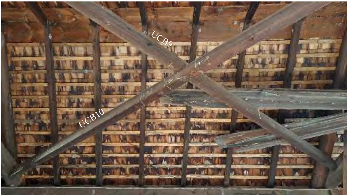
Figure 7-12: Upper cross braces UCB9 and UCB10. UCB9 is in fair condition.
