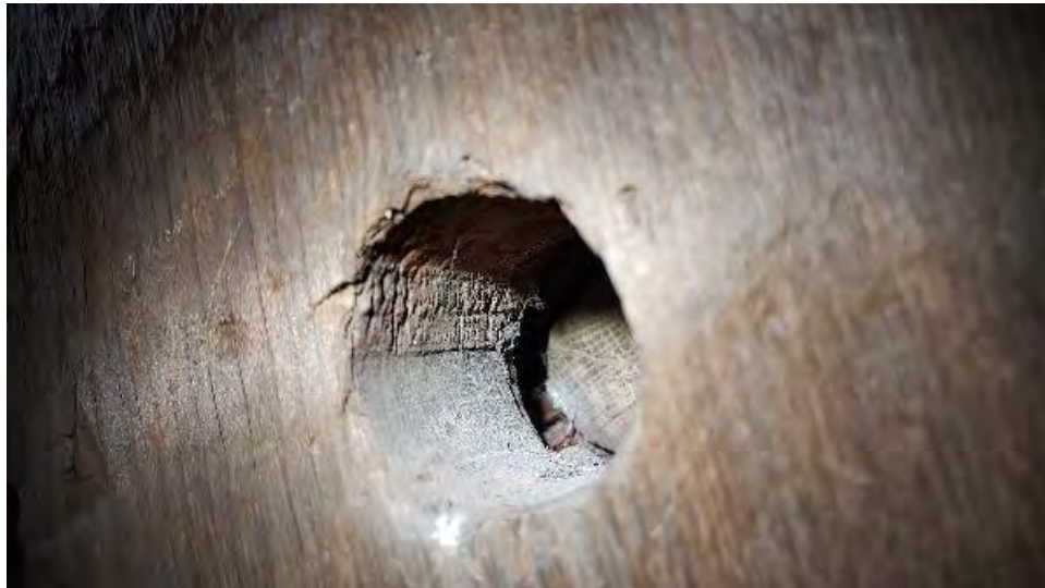
Figure 8-98: L4-7 is cracked through a row of dowels at the connection to L3-7. White surface fungi is seen on L3-7 above this connection. The top dowel does not penetrate through L4-7.
