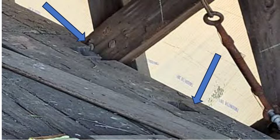
Figure 9-3: Floor decking Span 1, with 2 holes in Plank 1 on the north side.
