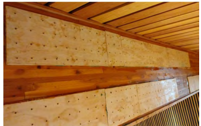
Retroshear™ panels to repair delaminated glulam timber beam.
