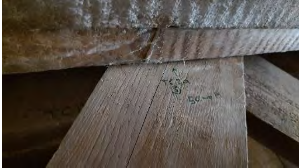
Figure 8-4: TC2A splice located 50-feet from post P1.
