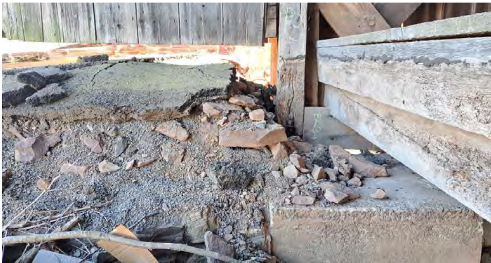
Figure 10-6: The mass concrete foundation at Ab1 appears to be undamaged.
