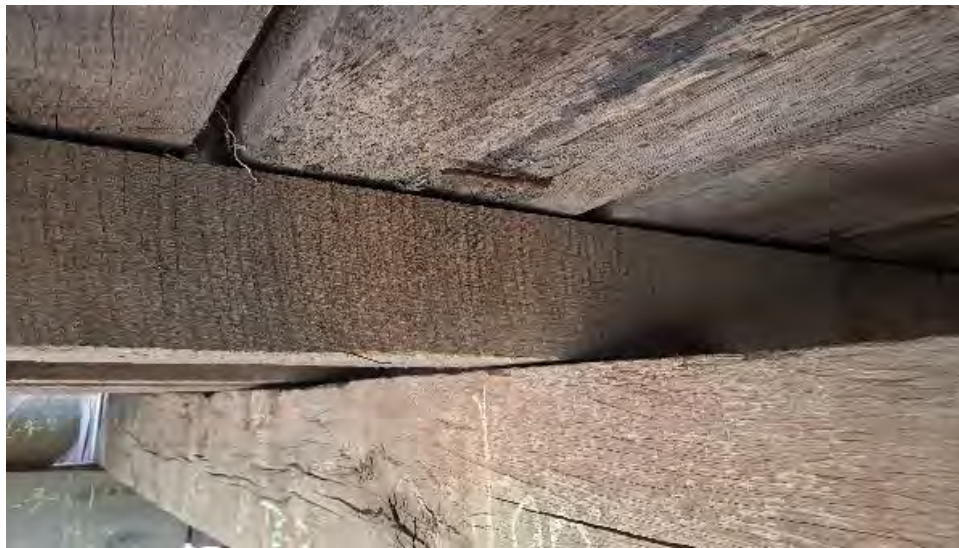
Figure 9-77: J1-4 is in fair condition.
