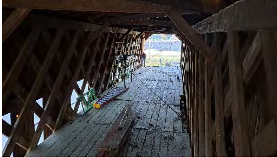
Figure 9-1: Top view of overall floor decking looking toward AB1.
