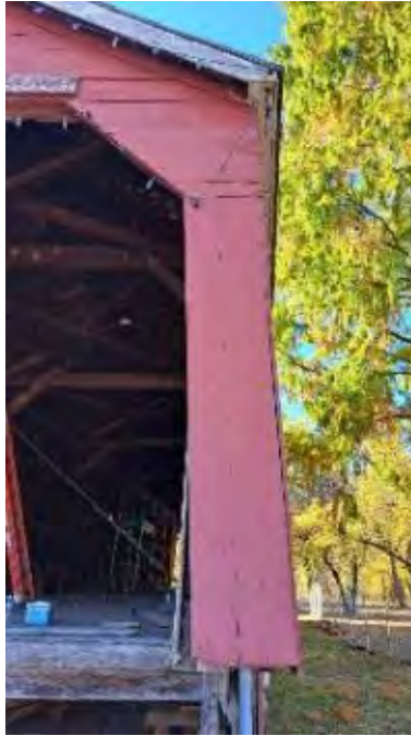
Figure 6-20: Abutment 1 North side front view of siding in fair condition.
