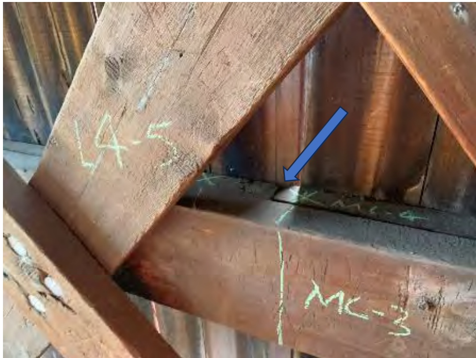
Figure 8-18: MC4 splice location behind lattice member LC4-5.
