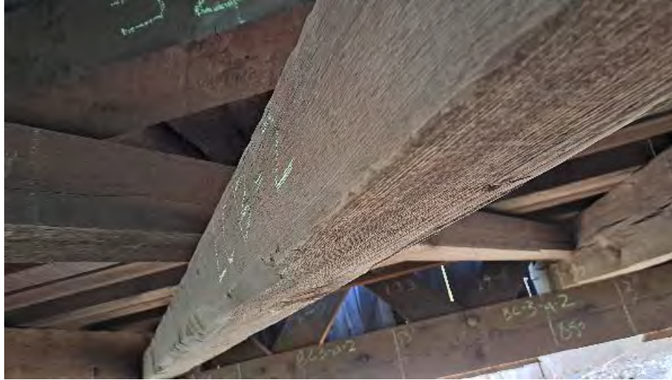
Figure 9-269: LCB-2 has some wane on its North side at midspan.
