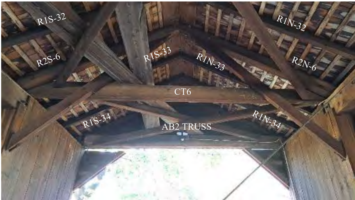
Figure 7-21: AB2 truss end, rafters seem to be in fair condition.
