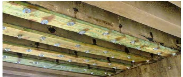
Treated Retroten installed on a series of bridge stringers.
