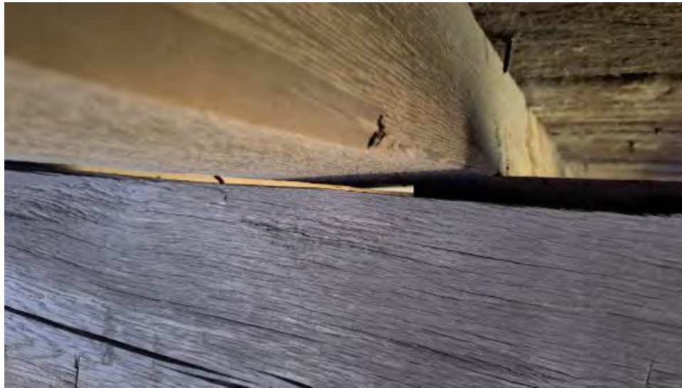
Figure 9-187: J7-5-N has partial bearing on packers at TB7 and TB8
