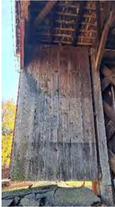
Figure 6-26: Abutment 1 South side wing wall internal view of siding.
