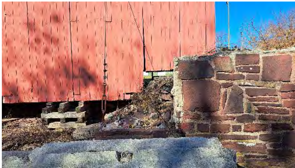
Figure 10-10: The backfilling at AB1 has receded and the asphalt surface is damaged for the full width of AB1.
