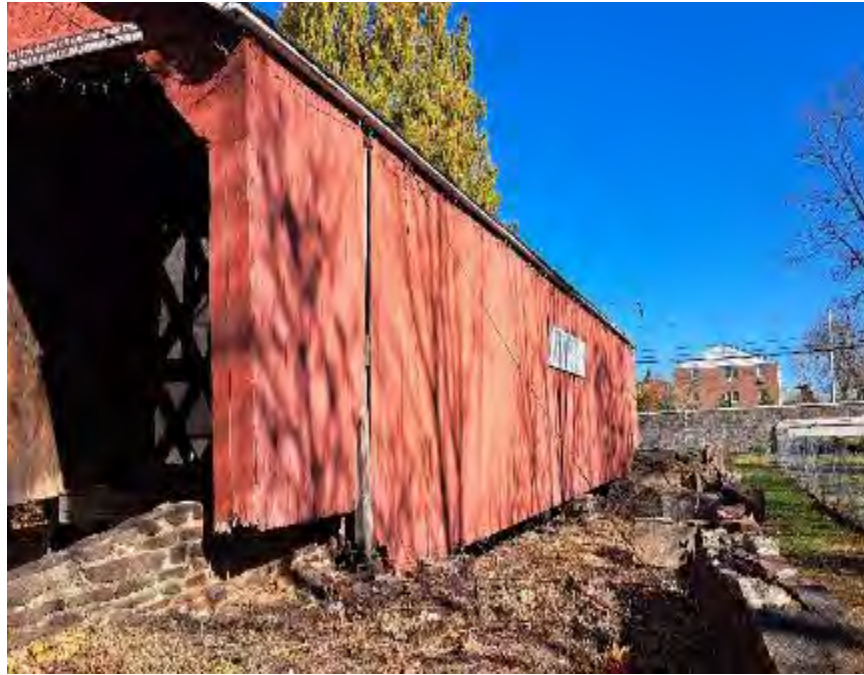
Figure 6-14: Siding on the South side.
