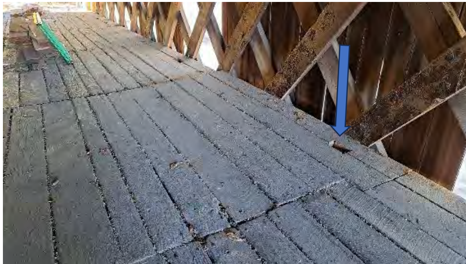
Figure 9-12: Floor decking Span 5, North side, with common hole in Planks 1 and 2.
