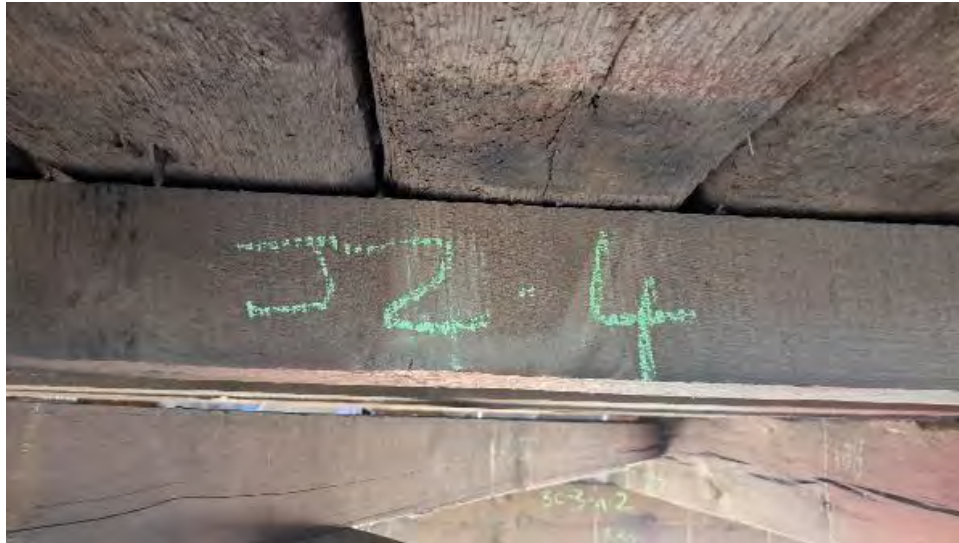
Figure 9-97: J2-4 is in fair condition.
