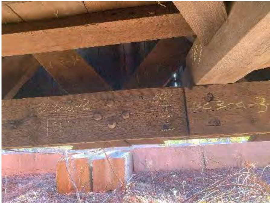
Figure 8-44: BC3A splice between Segment 2 and Segment 3.
