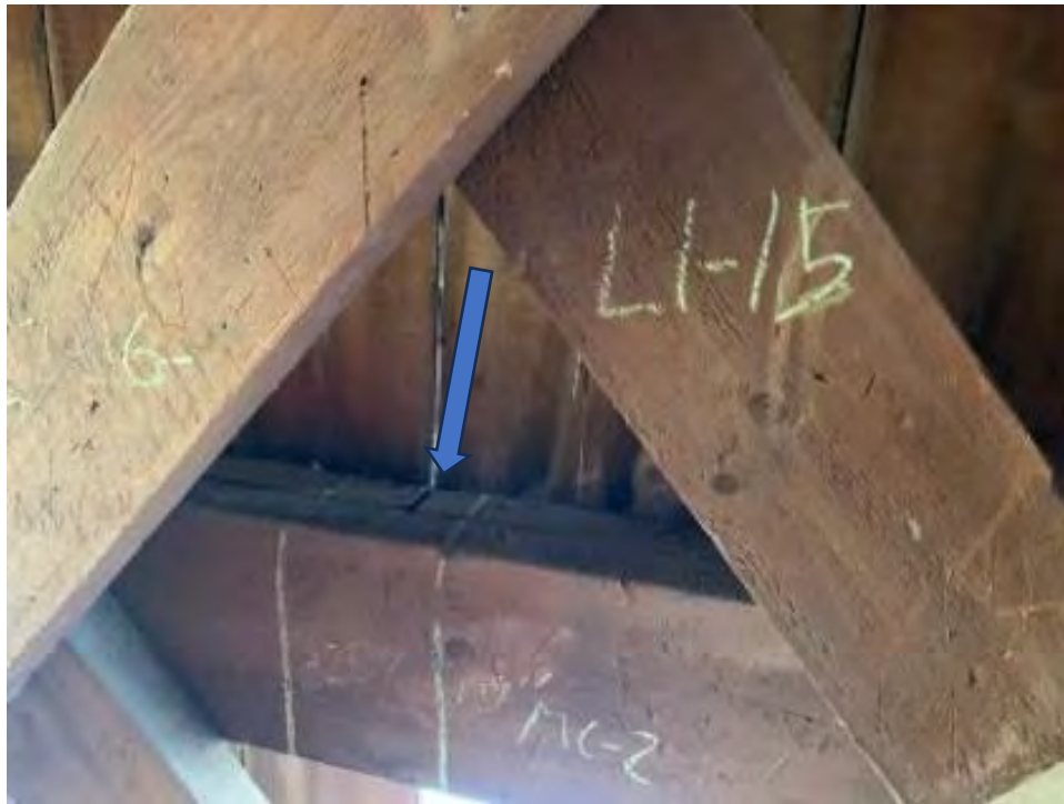
Figure 8-14: Middle chord MC1 showing a splice location behind MC2.
