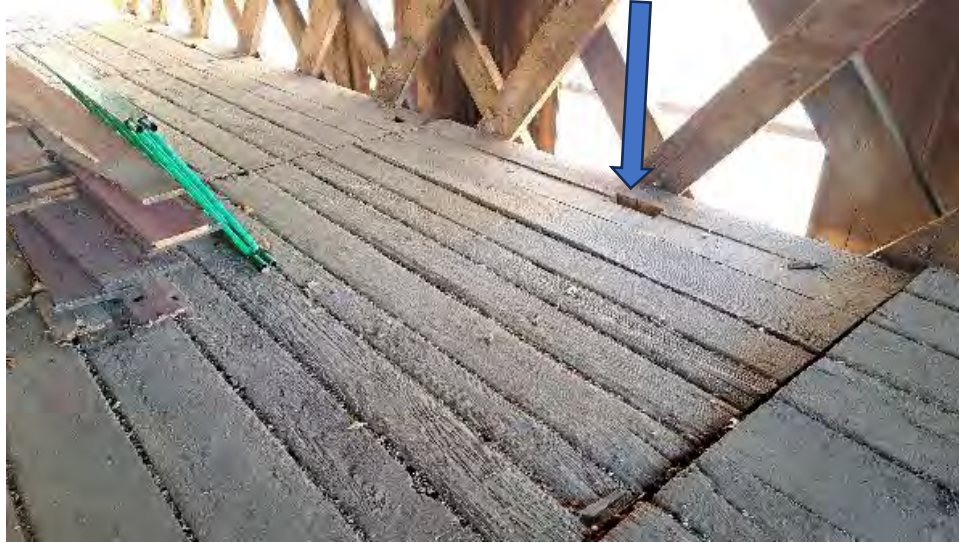
Figure 9-15: Floor decking Span 6, North side, with common hole in Planks 1 and 2.
