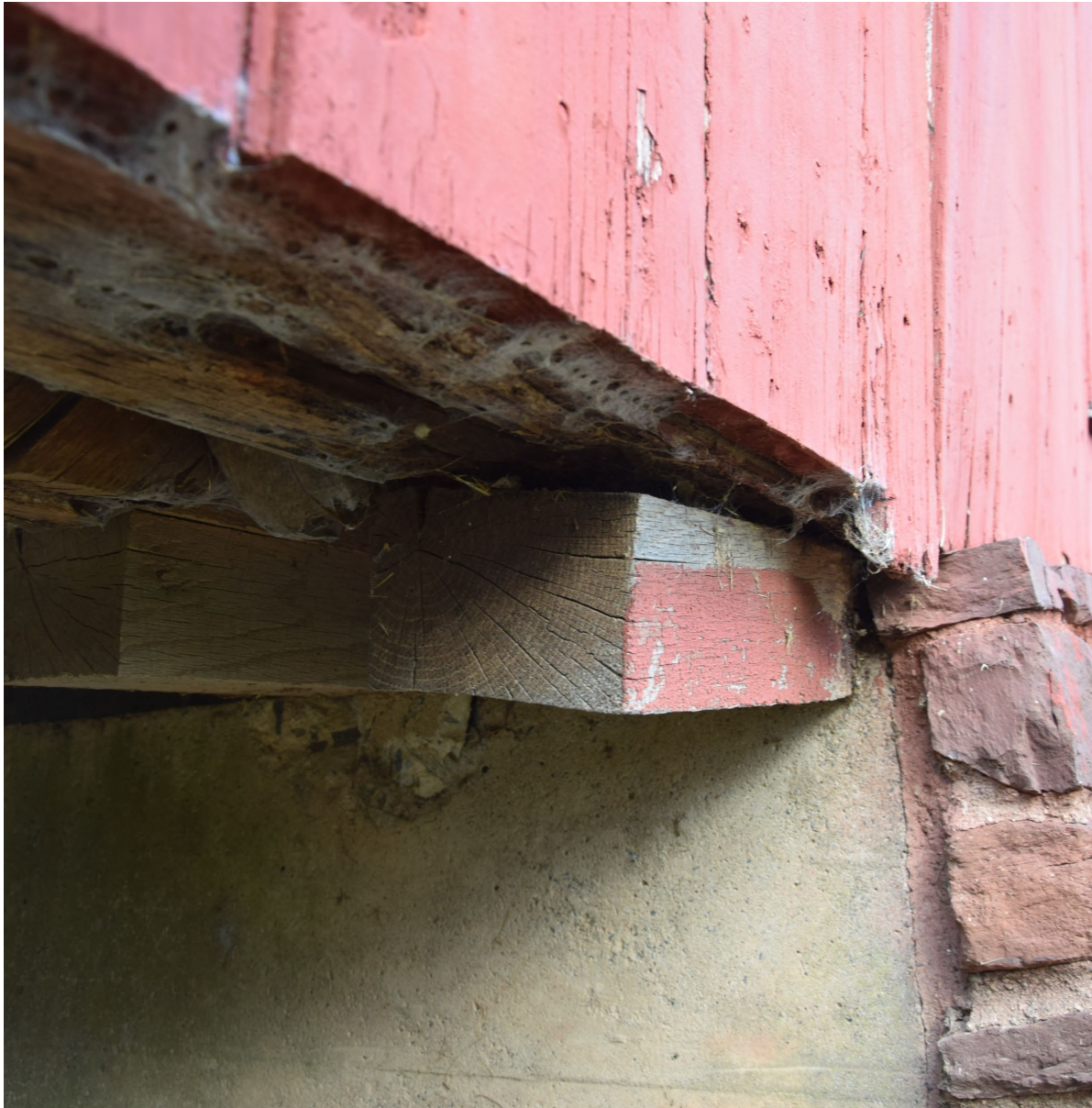
Bolster Block and Abutment Issue, Southeast Corner
