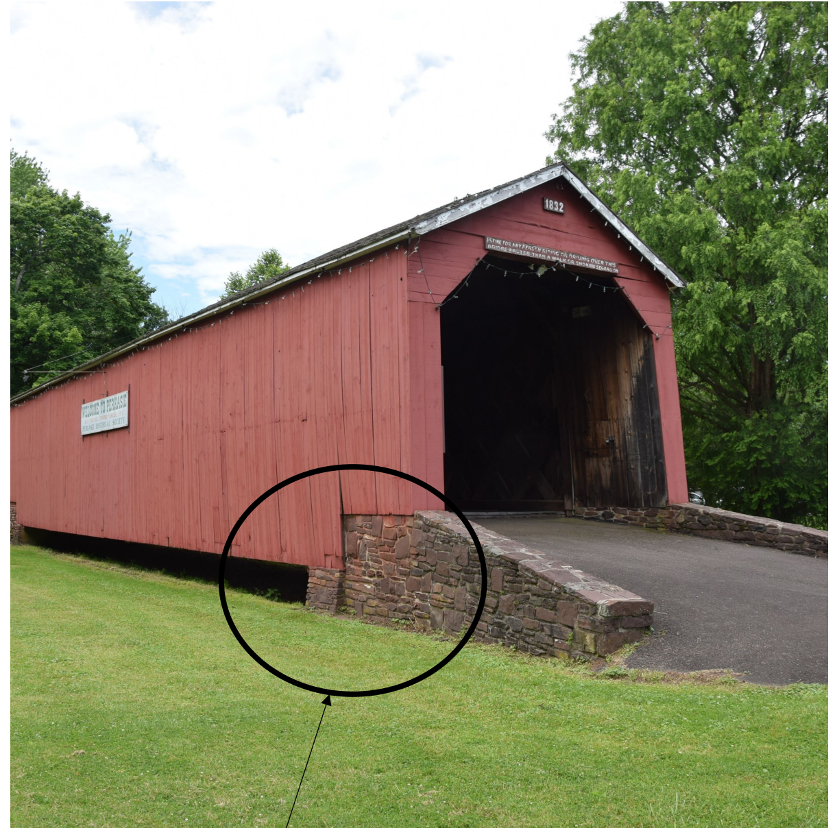
Bolster Block and Abutment Issue, Southeast Corner
